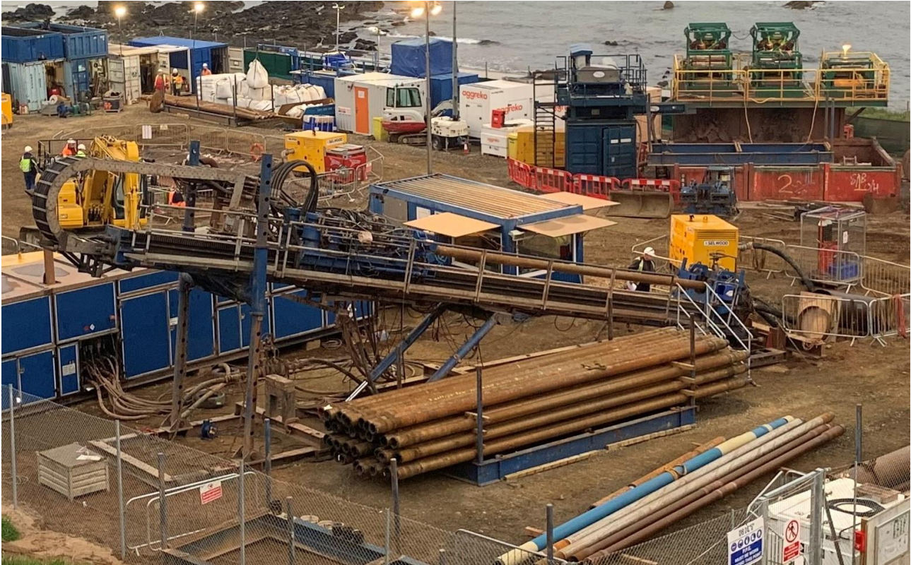
Image 9.1 Typical HDD Contractor Compound / Rig Setup
